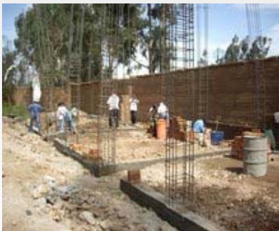
Foundation of the school
