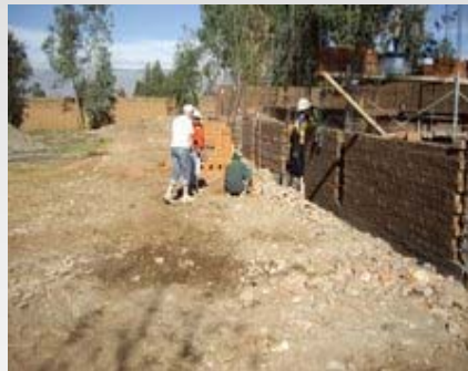
Now there are walls!
